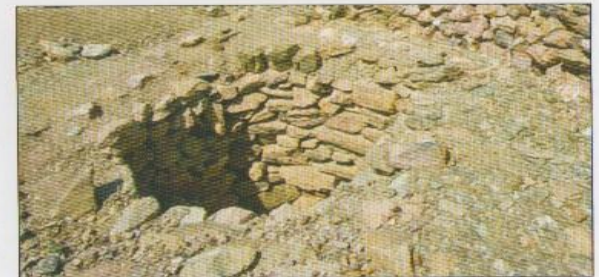
One of the wells affording access to the mines of Wadi Sikait
